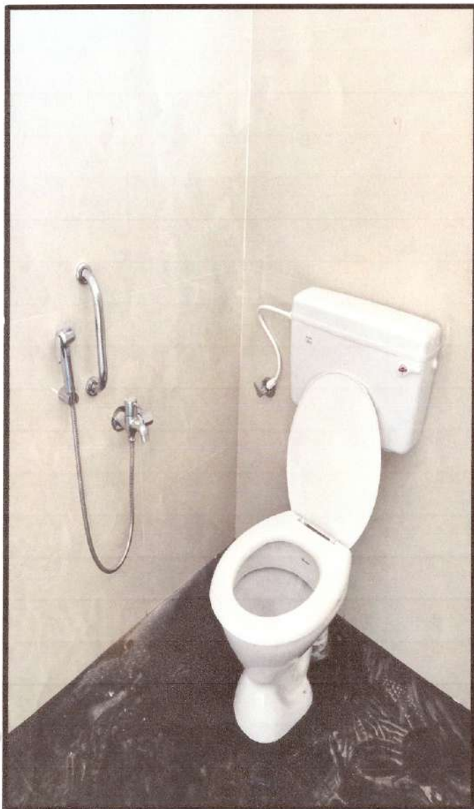
Divyang's Wash Room
